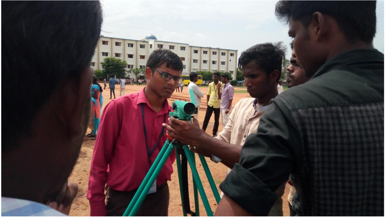
On-Site Training for the students on Foundation Marking
